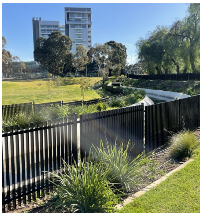
Concrete swale and fencing
