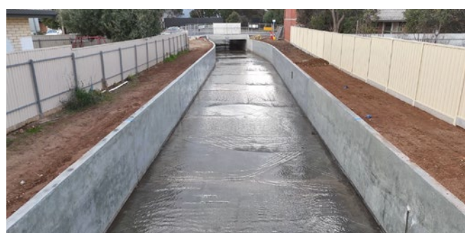
Channel construction through to completion
