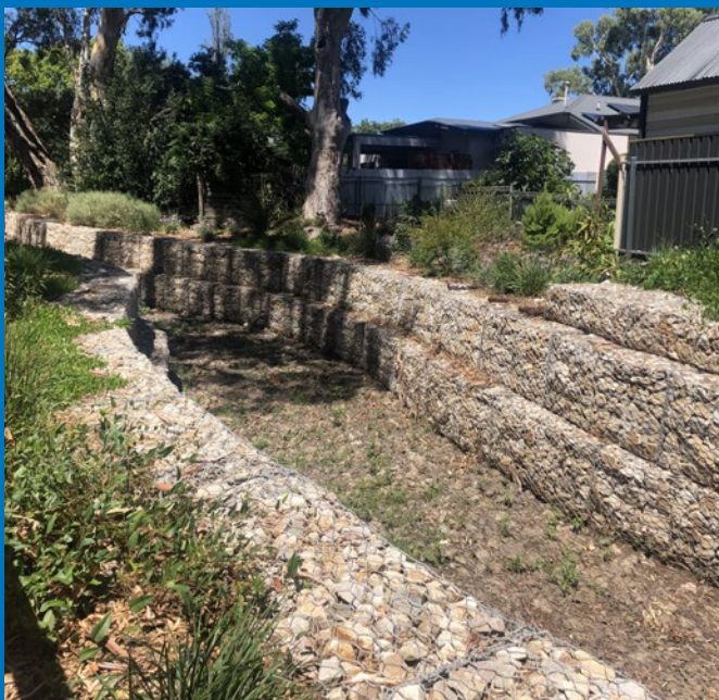
Rock filled gabions
